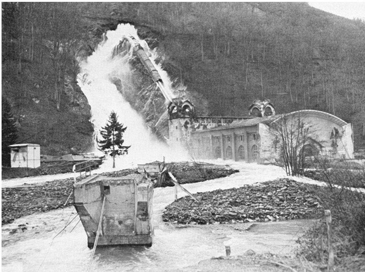
DAMAGED OBJECTIVE The Hydro- electric power station at Heimbach was captured intact but the Germans had blown the pressure pipe leading from the Urft dam. NATIONAL ARCHIVES
